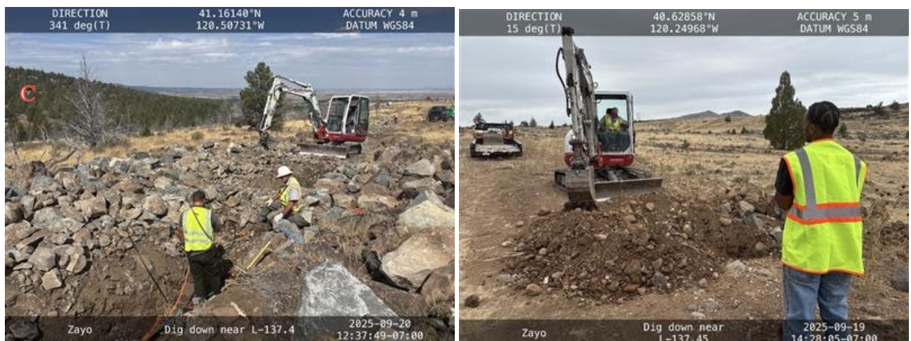
Figure 7. View of typical dig down operations in Northern Area (Lassen County).
