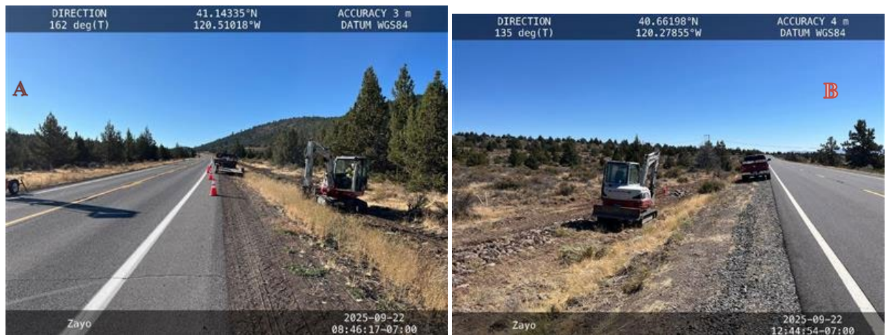
Figure 6. View of typical dig down operations in Northern Area (Lassen County).
