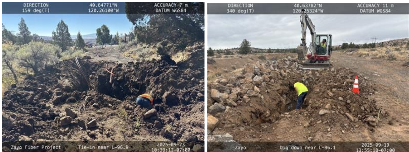
Figure 1. View of tie-in/dig-down operations in Central Area (Lassen County).
